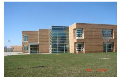
White Oaks Elementary School is a 2-story steel frame building built in 2001. The building's exterior components consisted of several types of wall and roof systems. The majority of the roofs were designed to receive a low-slope modified bitumen roofing system with tapered insulation. Two of the roofs were standing seam metal roofs.
